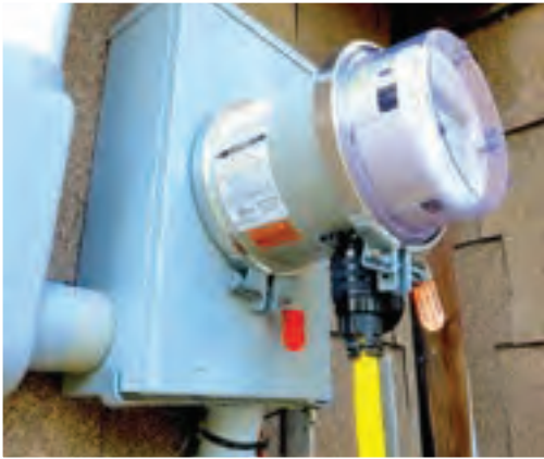
Photo of GenerLink transfer switch and standby unit on a dairy farm from Sommers Generators
