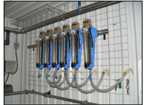
Fig. 25. Milk meters need extra cleaning
