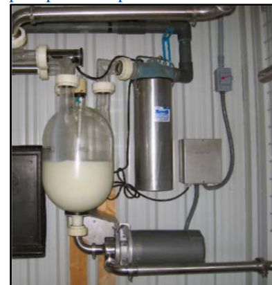
Fig. 33. Receiver jar with milk pump and trap
