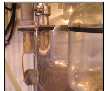
Fig. 39. Check sanitary trap for cleanliness
